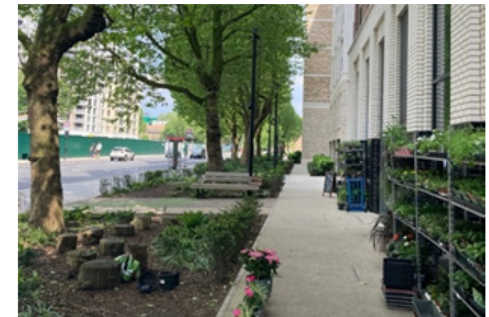
Figure 8.30: SuDS incorporated within Heygate Street, Southwark
