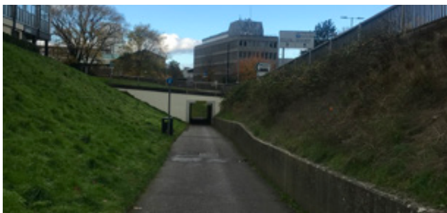
Figure 7.4: Subway on approach to the town centre from the east with Easthampstead House in the background
