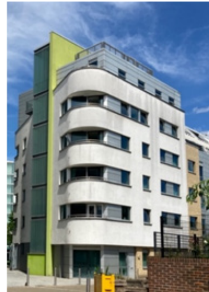
Figure 8.14: Corner articulation gives the opportunity to address two streets creating a marker
