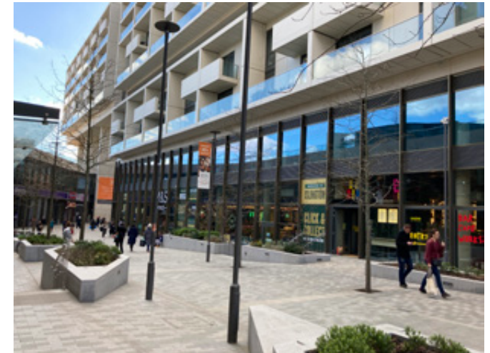
Figure 5.45: City North Place, Finsbury Park
