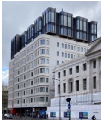
Figure 7.21: Easthampstead House can be refurbished and extended at roof level with terraces providing long distance views, example: ex Camden Council Office, London
